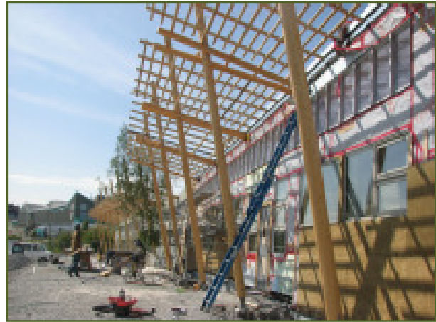
Kalemi Dene School under construction in N'Dilo
